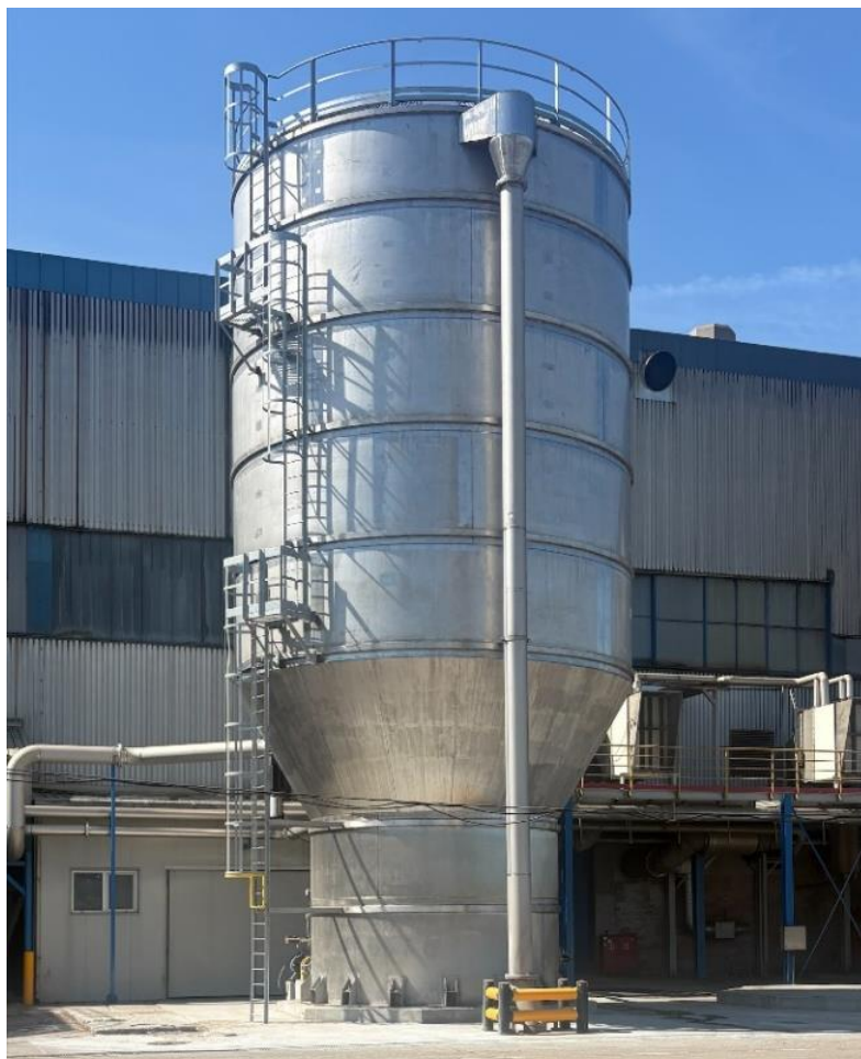
Figure 3. 600 m 3 screen water tank in SWB
