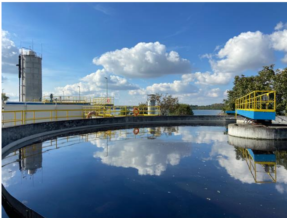
Figure 6. View of a section of the WWTP from the secondary clarifier
